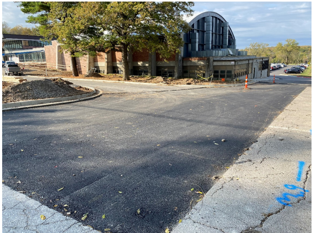
Main entrance base coat (below)
